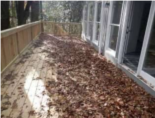
Photo 14-4 (R) side view of deck
