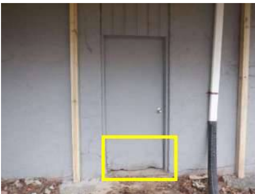
Photo 25-1 Crawlspace door entry
