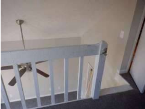
Photo 24-1 (R) living area guardrail
