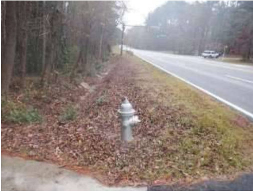
Photo 8-1 The right side of Hwy 92 N fire hydrant
