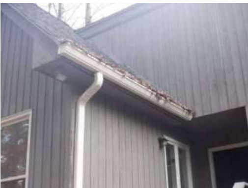
Photo 28-1 clogged gutter
