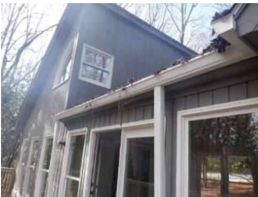
Photo 28-2 clogged gutter
