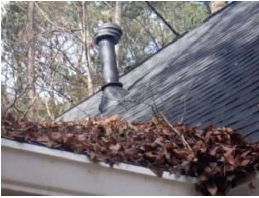
Photo 28-3 clogged gutter
