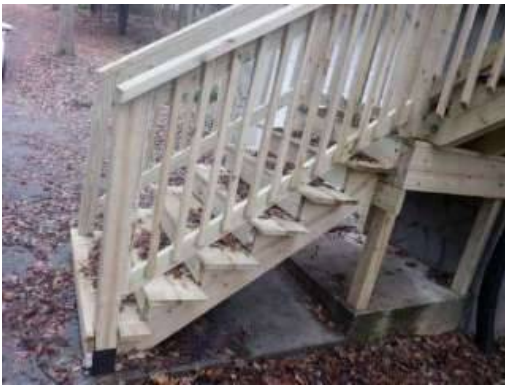
Photo 9-1 (R) side of Deck stairway
