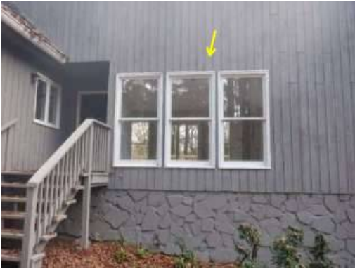
Photo 16-1 Front three windows
