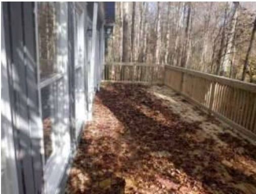
Photo 14-5 (L) side view of Deck
